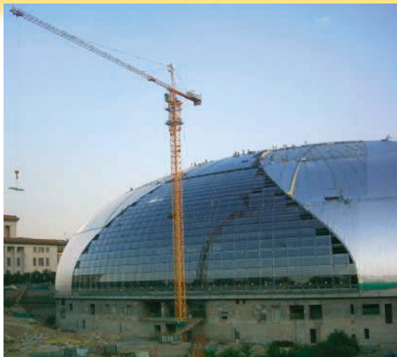
Operatic nanoscience. Now under construction in Beijing, China’s new National Opera Hall features self-cleaning glass coated with a film of photocatalytic nanoparticles that can break down dirt.
